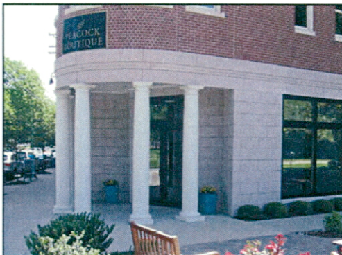
Building corner entry with columns, recessed entry, and change of material.
