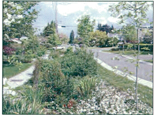
Raingarden between sidewalk and adjacent roadway.
