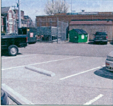
Permeable asphalt paving.
