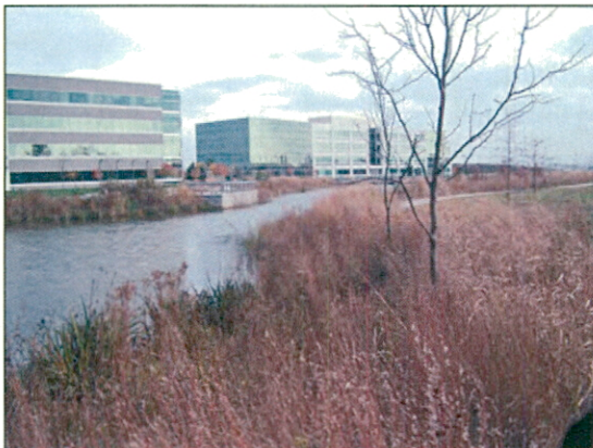
An example of regional / shared stormwater detention that is also an amenity.
