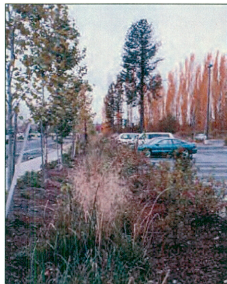
Stormwater filtration within a parking lot.
