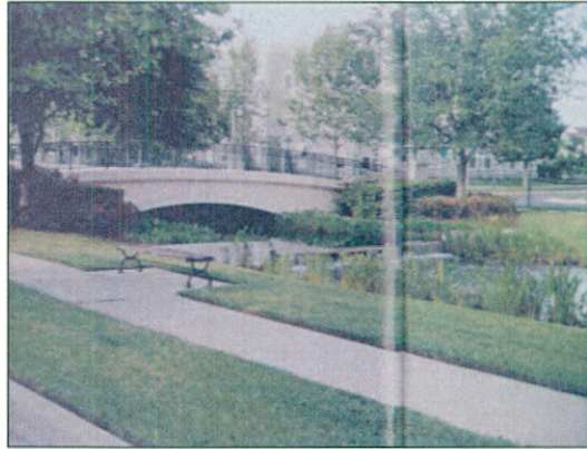
Stormwater facility that doubles as an amenity,
