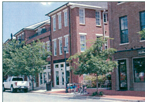
New commercial mixed-use "village style" development.
